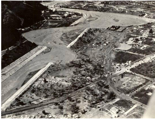
Flooding of Los Angeles River along Victory Blvd.
