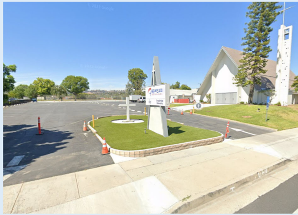
Site 18: Former Lutheran Church
