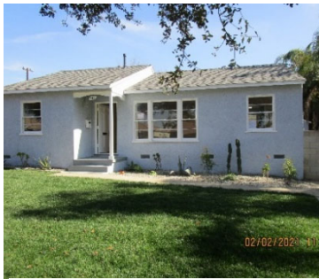
Code enforcement efforts leading to housing repairs.
